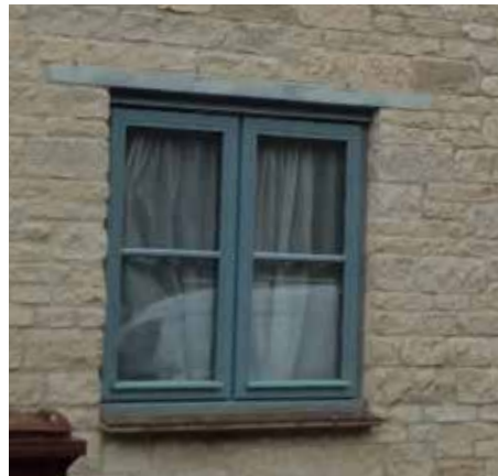
Casement window flush with wall, Bletchingdon
