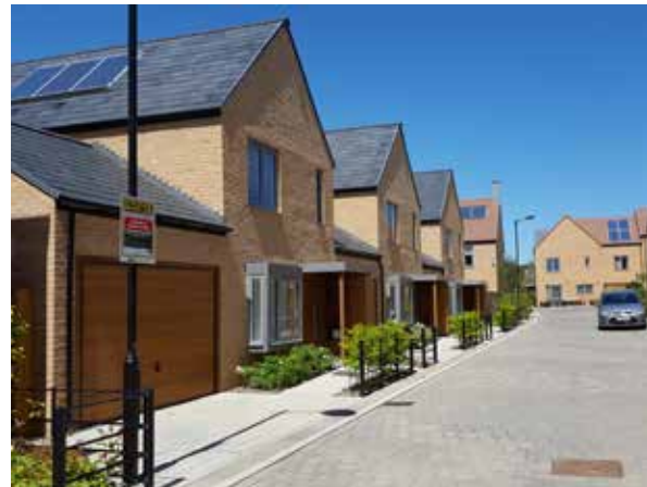
Photovoltaic panels, Trumpington Meadows, Cambridge
