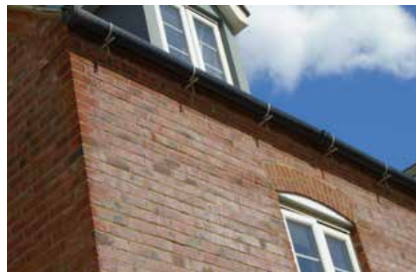
Guttering, South West Bicester
