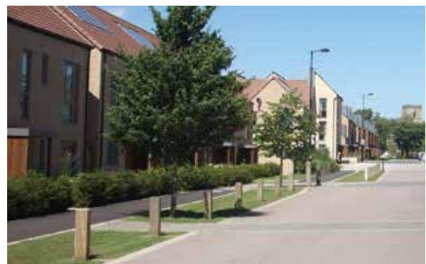
Incorporating SuDS along kerbside, Trumpington Meadows, Cambridge
